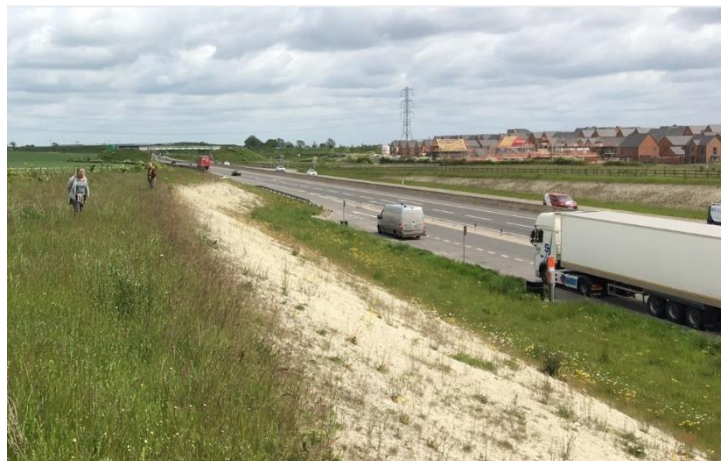
Surveying the chalk cutting, May 2023
