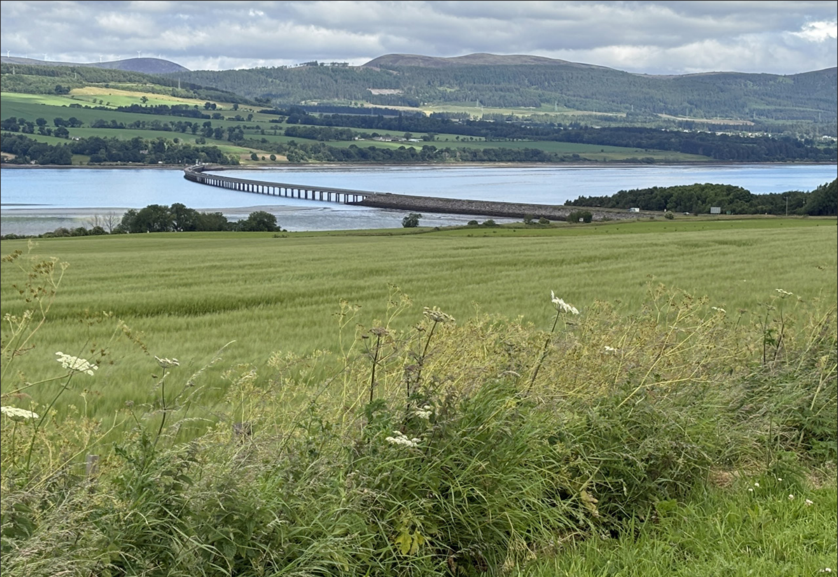
Bridge 2: Cromarty Firth, 1,464m
